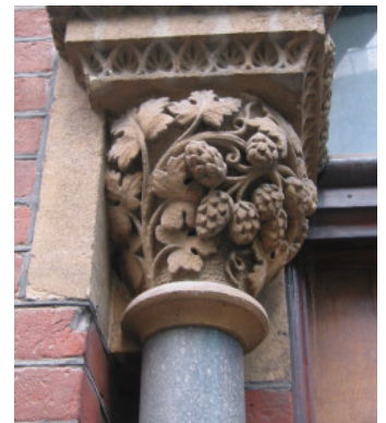
This hops and barley detail is still visible on the old Cannon's Brewery building on St John Street.
