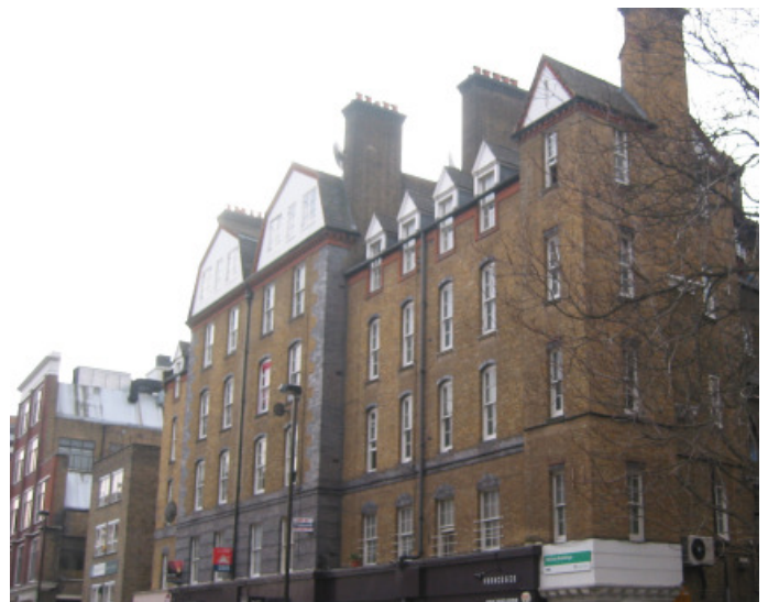
The Mallory Buildings, St John Street, built by the London County Council 1906-07
